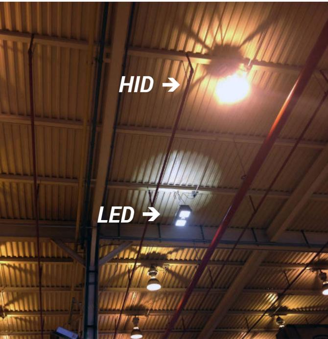
Weldbend's LED retrofit consisted of Verde Solutions replacing 987 HID highbays with 987 LED highbays. There was a significant reduction in maintenance and replacement costs going from the HID rated life of 10,000 hours to the LED rated life of 50,000 hours. Weldbend would have to replace their existing HID highbays 5 times over the lifetime of just one Verde Industrial Highbay.
