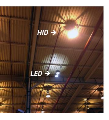
Weldbend's LED retrofit consisted of Verde Solutions replacing 987 HID highbays with 987 LED highbays. There was a significant reduction in maintenance and replacement costs going from the HID rated life of 10,000 hours to the LED rated life of 50,000 hours. Weldbend would have to replace their existing HID highbays 5 times over the lifetime of just one Verde Industrial Highbay.
